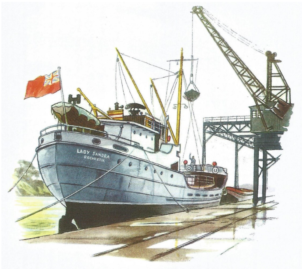
China clay from Cornwall being unloaded into bunkers
